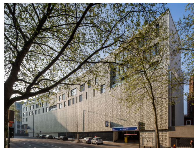
Fig.6: Magnus 31 © Wilkin & Hanrath Bauphasen
