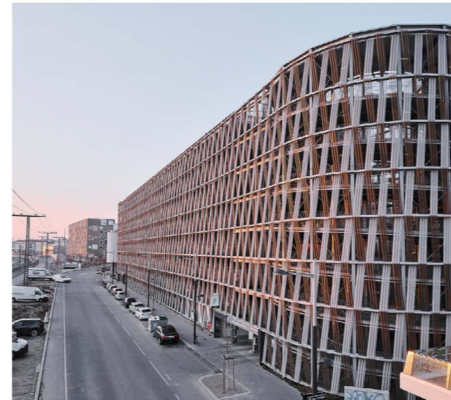
Fig. 22: Multi-storey car park main station Vienna © David Schreyer
