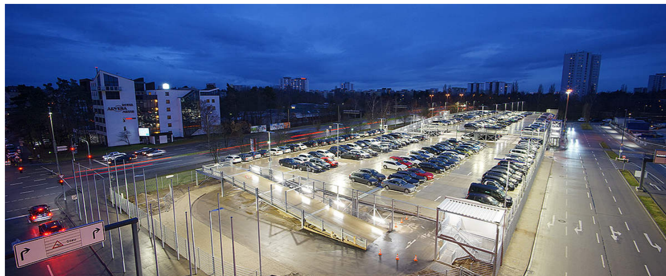
Fig. 24: Christmann + Pfeifer Construction GmbH & Co. KG, Nuremberg car park built with the Preflex® system
