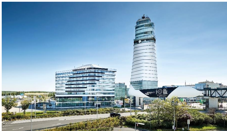
Abbildung 8: Office Park 4, Vienna International Airport, FWAG
