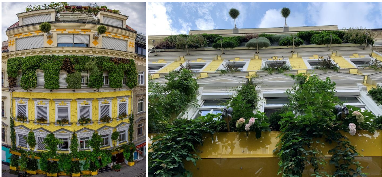
Figure 13: Combination of different facade greening systems, Hannovergasse Vienna
